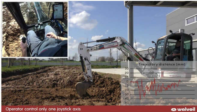
Excavator activity with Operating Assistance System
